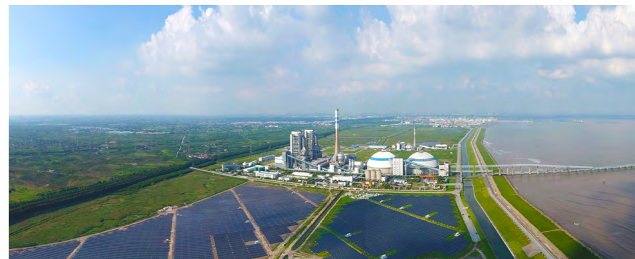
国家电投上海漕泾电厂 SPIC Caojing Power Plant in Shanghai
